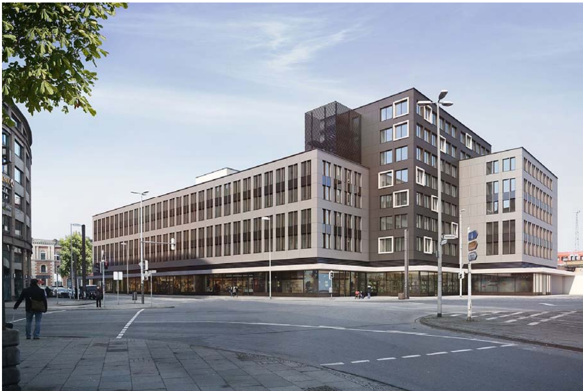
Photo 1: The building complex at Joachimstraße 8 in Hanover (© Architekturbüro Schulze & Partner, Hanover)
