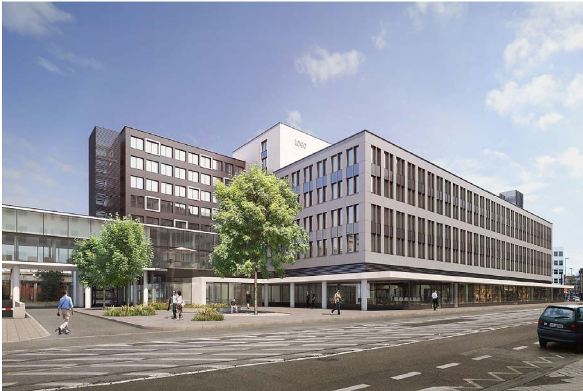
Photo 2: The building complex is connected to the Ernst August Carrée center by means of a gallery (on the left in the photo) (© Architekturbüro Schulze & Partner, Hanover)
